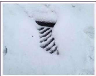
**Culverts:** Another common conveyance structure which can cause flooding are obstructed road and driveway culverts. Drainage systems rely on many drainage structures to convey water safely downstream. An obstruction at any of these points can back up water far upstream, impacting many property owners. If you suspect a culvert is blocked, the appropriate utility owner should be contacted.
